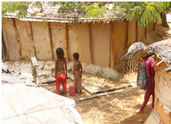
Type 6: Mud wall, bamboo and tarpuline for roof
