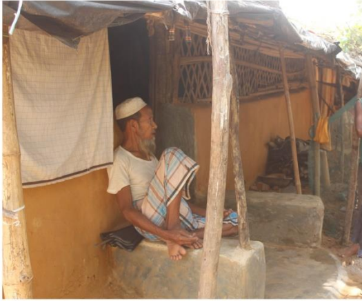
Type 9: Mud house with concrete plinth
