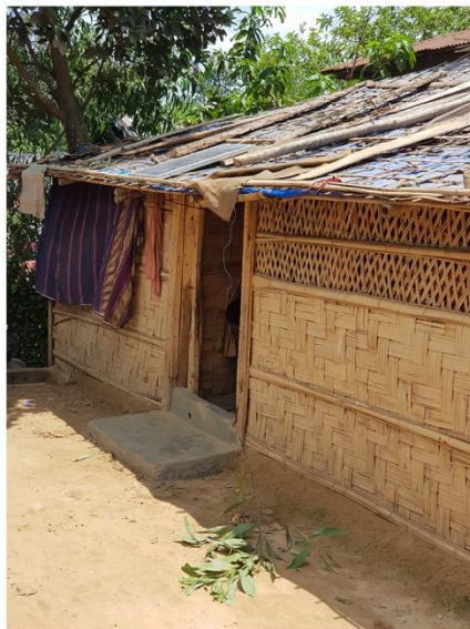
Type 3: Bamboo mesh for wall, tarpuline roof
